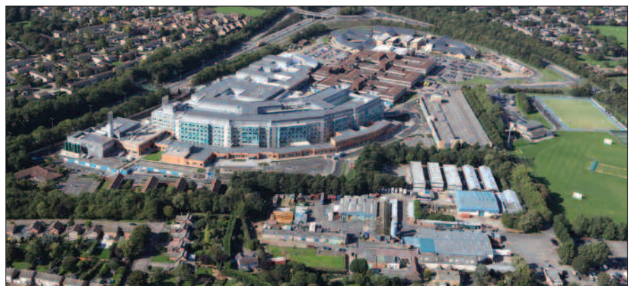
The site of the new Peterborough City Hospital, where System Hygienics recently completed a major pre-commission clean.
