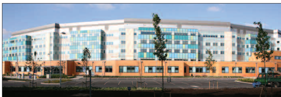
The ventilation system serves the entire 96,000 m 2 hospital building at the new Peterborough City Hospital, including intensive care units (ICUs), theatres, wards, technical rooms, canteens, and cleaning cupboards.
