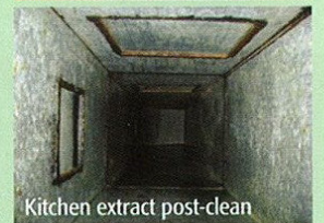
Kitchen extract post-clean
