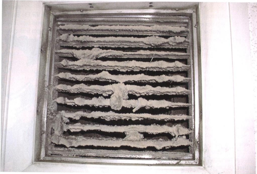
The picture above shows ventilation ductwork before cleaning, while the picture below was taken post-clean. Accumulation of dust and moisture within HVAC systems increases the risk for the spread of airborne pathogens, so regular cleaning and maintenance should be carried out to guard against this
