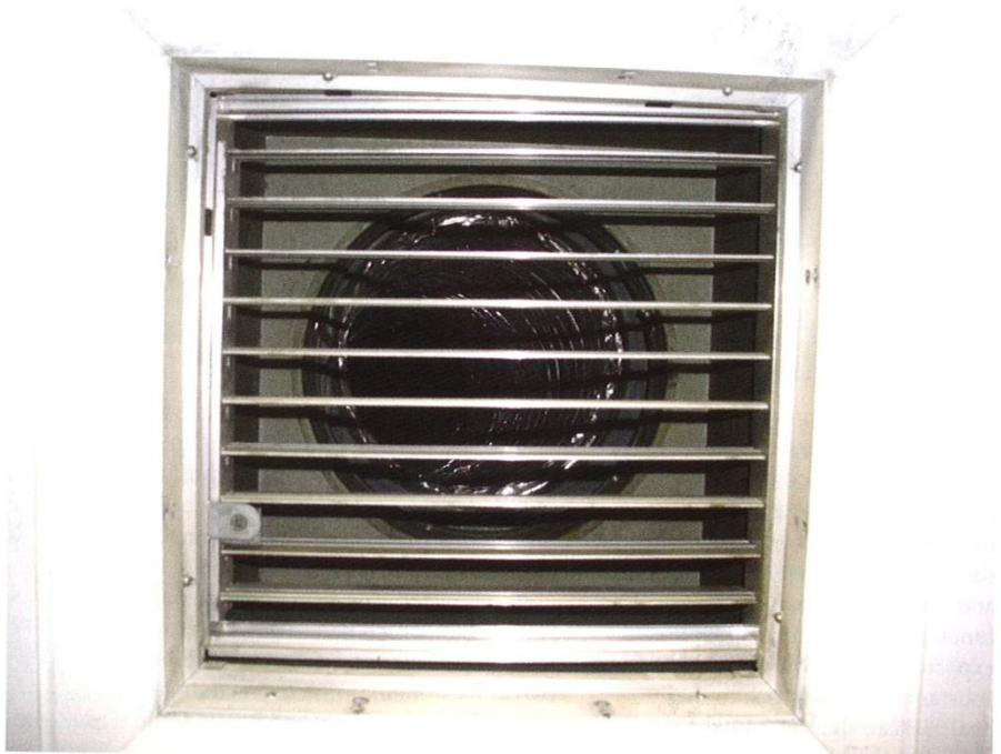
The picture above shows ventilation ductwork before cleaning, while the picture below was taken post-clean. Accumulation of dust and moisture within HVAC systems increases the risk for the spread of airborne pathogens, so regular cleaning and maintenance should be carried out to guard against this
