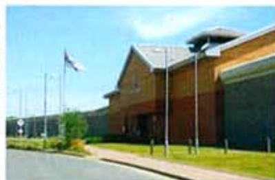
Large-scale cleaning of ductwork in HM Prison Doncaster has been completed by System Hygienics.
